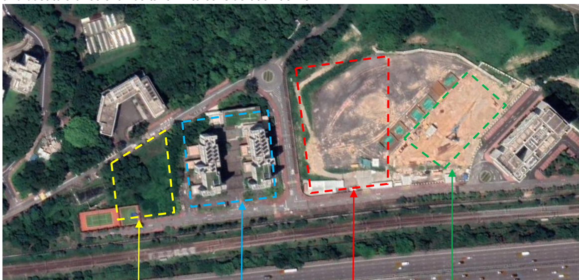
New hostel for postgraduate students Jockey Club Postgraduate Hall 2&3 New Teaching-Research Complex New laboratory building
